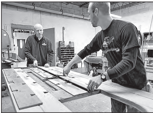
ABOVE: Sean Clarke, left, and Jeremy Mills replace damaged panels on the Reichs' front door.
